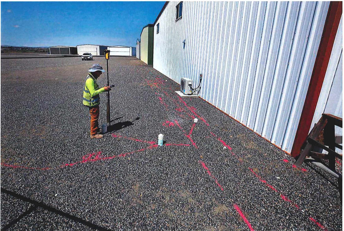
Mark Villa, of Geophysical Survey in Kennewick, maps out underground lines he marked with paint by using ground penetrating radar inside the fenced hangar area at the Port of Benton's Richland Airport. Bob Brawdy bbrawdy@tricityherald.com
